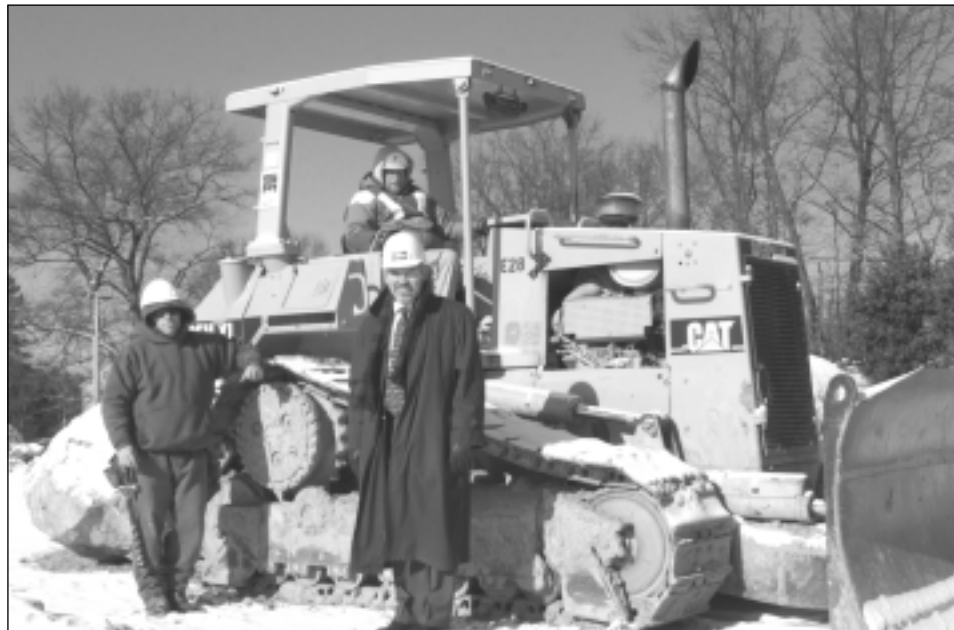
Frederic Mulligan (in trench coat) with Cutler crew members at a job site on Worcester's East Mountain St. Left to right: Jerry Simmer (standing) Terry Simmer (in cab) and Mulligan.
